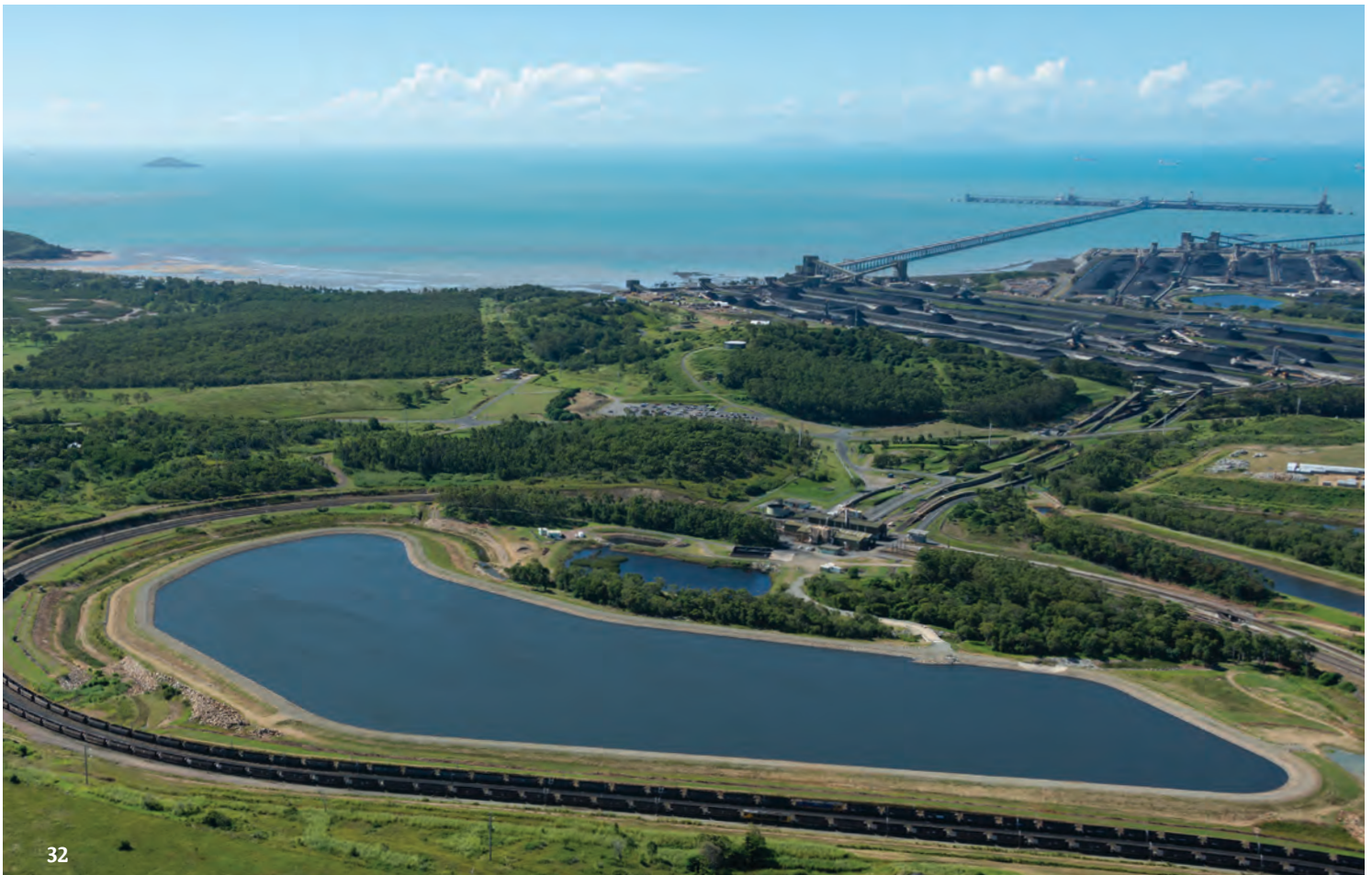
Aerial view from Rail Loop Dam, including DBCT onshore and offshore infrastructure, Hay Point Coal Terminal (right) and surrounding environment.
